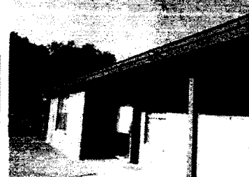
Rear entry view
