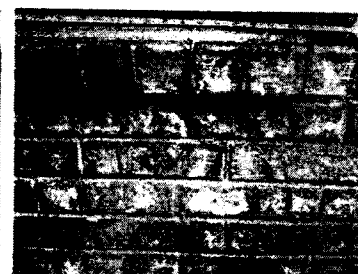
Brick/Mortar cracking
