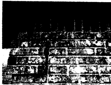
Brick/Mortar cracking
